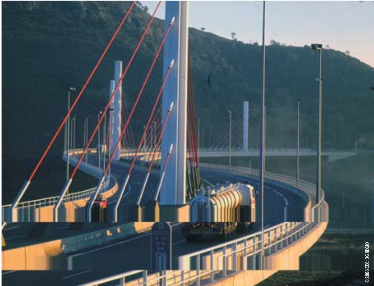
Bridge on new Bilbao to Santander motorway, near Las Arenas, Basque Country (Spain)
