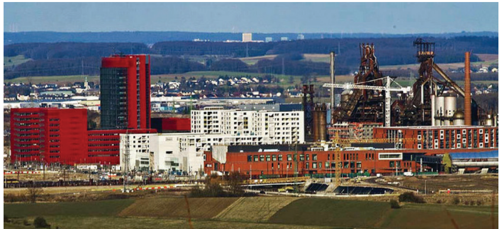
The site of Eco-Cité d'Esch-Belval in the south of Luxembourg
